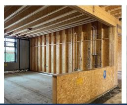
**Sprinkler System:** The first-fix installation of the sprinkler system is underway on the ground floor, including supporting bracketry for the pipework.
